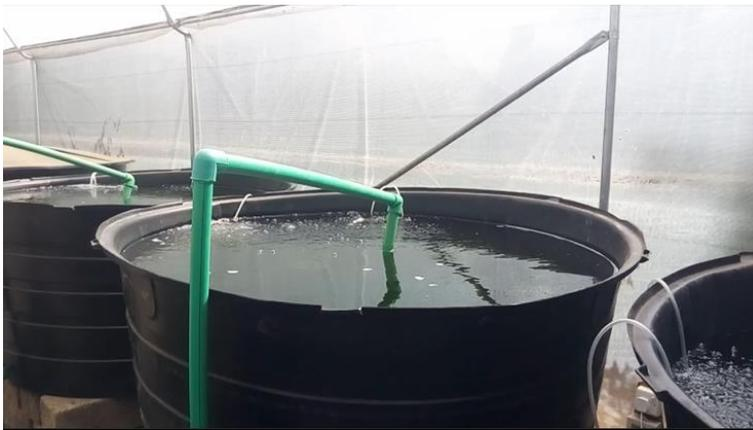
Figure 3.3: The production tanks showing return water pipes and aerator leads pumping air into the water.
